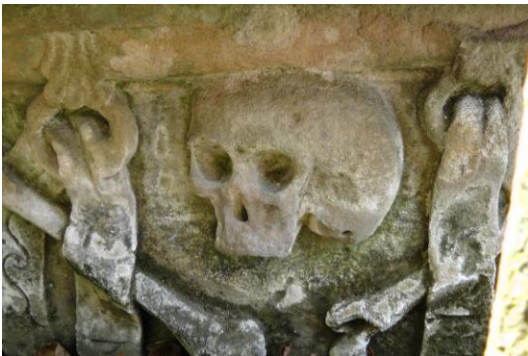
Some of the exceptional work by masons at Cullen
