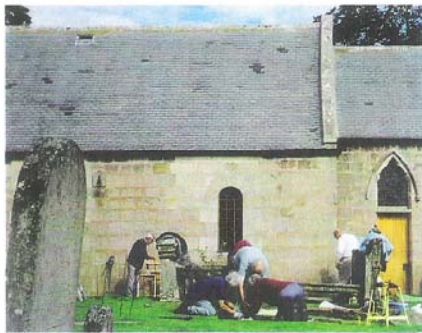
Work in progress, Birnie Churchyard, September 2006 (courtesy Betty Willsher)
